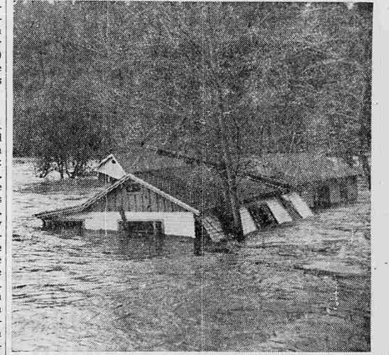
DECEMBER FLOODS CREATE WIDE DESTRUCTION
