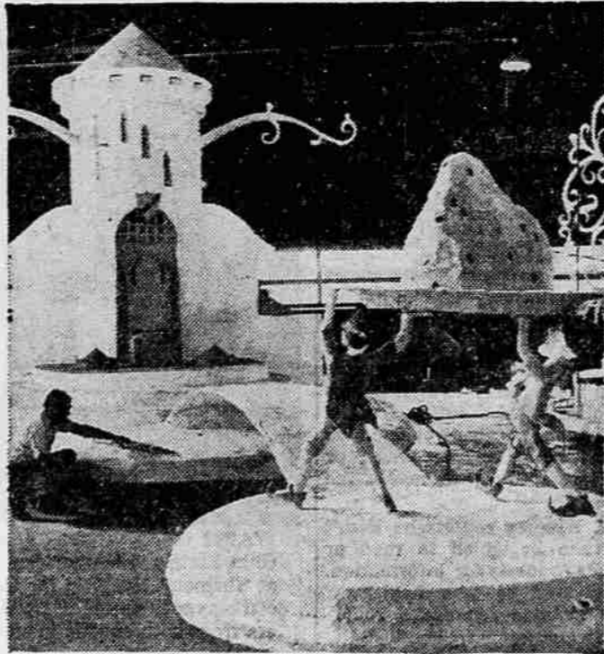
PRESENT-DAY FLOATS are products of skilled artists, designers and craftsmen. The metal frame is covered with chicken wire, sprayed with plastic "cocooning," then covered with flowers.
