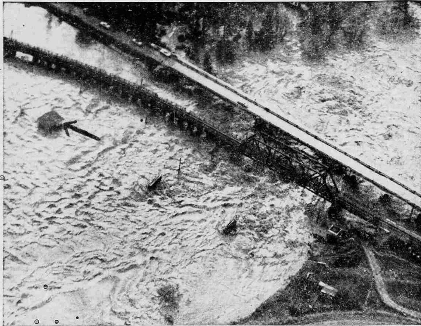
SCENE OF RESCUE —This dramatic aerial photo, taken by Carl Landis of the Landis-Shangle studio from a Mercy Flights plane, shows the old highway bridge and the railroad bridge across the Rogue river at Gold Hill, near the home of Barney Governor who was rescued from his house yesterday afternoon after being surrounded by surging flood waters for more than 12 hours. The arrow at the left of the picture shows the
