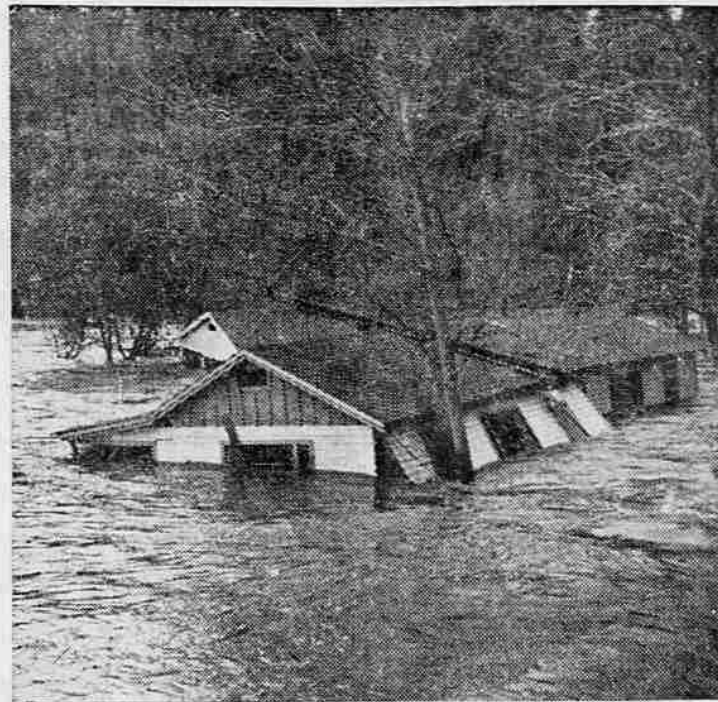
RESORT A SHAMBLES —Riffles on the Rogue, a resort on the Rogue river above Shady Cove, was virtually wiped out by high water Thursday morning. It is shown soon after the flood crest passed in the picture above, taken by Don Hinson of Eagle Point.
