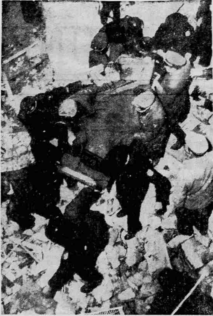
GERMAN APARTMENT HOUSE EXPLODES — Rescuers carry injured occupant from debris of a new five-story apartment house in Frankfurt which collapsed after an explosion. Police estimated 25 to 28 of 35 persons believed in the building were killed. Seven were hospitalized with injuries. U. S. soldiers and equipment were rushed to the scene to aid police in digging victims from the wreckage.
