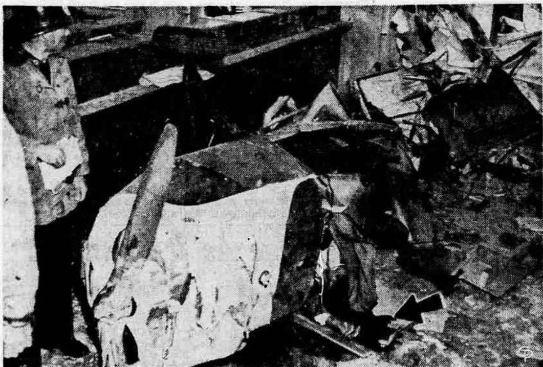
WRECKAGE LITTERS interior of Los Angeles Bank of America branch after light plane flown by employe let out of his job just the day before smashed into building. Witnesses said it appeared the pilot, Benjamin Fauth, 29, deliberately aimed his aircraft at the bank building. He was instantly killed, and one bank employe was injured. (International)
