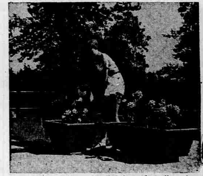
TEXTURE ONE ELEVEN PLANTER boxes for patio or terrace, are a lot easier to make than they look. The difficult custom-built effect shown incorporated in the design does not involve fancy carpentry. It is achieved by use of grooved fir plywood called Texture One-Eleven. This is a 3/8" panel manufactured with 100% waterproof glue with deep grooves on the panel face. It comes with the grooves 2" or 4" o.c. The boxes can be made simply by cutting the panels to the size required and assembling them with the trim.
