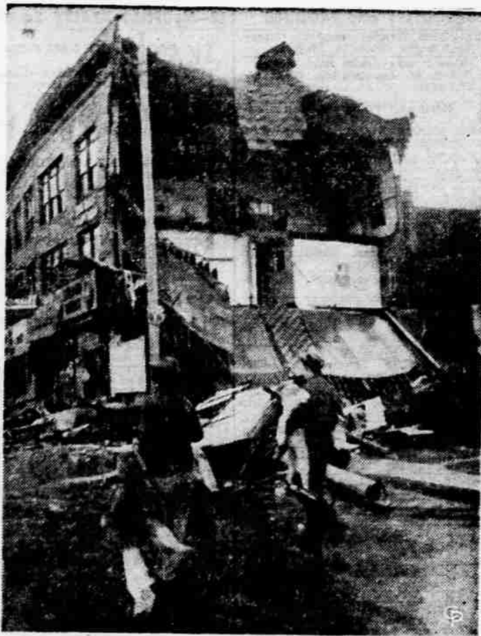
RACING FROM CAVE-IN, residents of Norwalk, Conn., seek shelter as flood waters undermine buildings, rendering thousands homeless. Building at right was collapsing as torrent ripped through foundations in wake of storm. (International)
