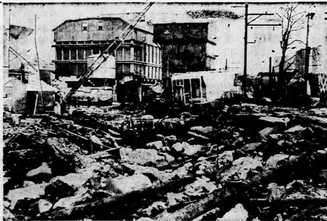
RESULT OF RAMPAGING WATERS —Flood-strwn debris covers the New York, New Haven & Hartford freight yards in Norwalk, Conn., after the ravaging waters receded. Connecticut was the hardest hit of seven northeastern states from hurricanes and floods that took 50 lives. More than 25,000 persons were left homeless and damage was estimated at 500 million dollars.
