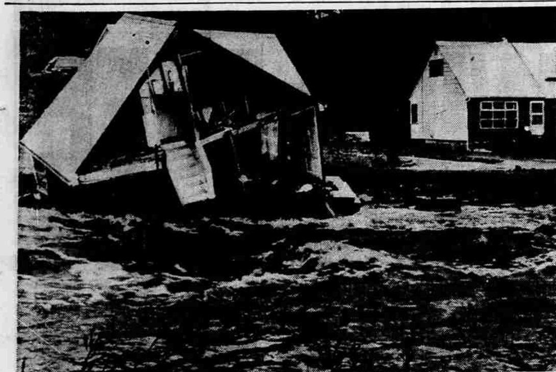
FLOOD CLAIMS HOME —With one of its sides torn away, a house begins to topple into the raging Byram River in Greenwich, Conn., as the normally quiet stream undercuts its banks. Flood waters from heavy rains have driven thousands from their homes and caused millions of dollars' damage.
