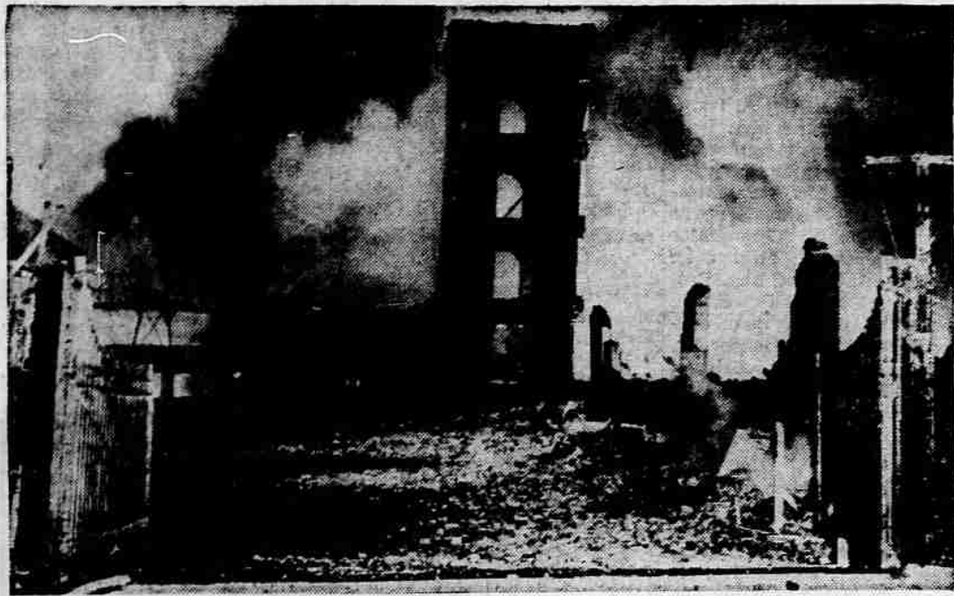
GATES TO HELL —Looking like the "Gates to Hell" describes this scene at the five-million-dollar fire that destroyed mills in Manville, R. I. Civil defense and Red Cross units were called to the huge state alarm fire.
