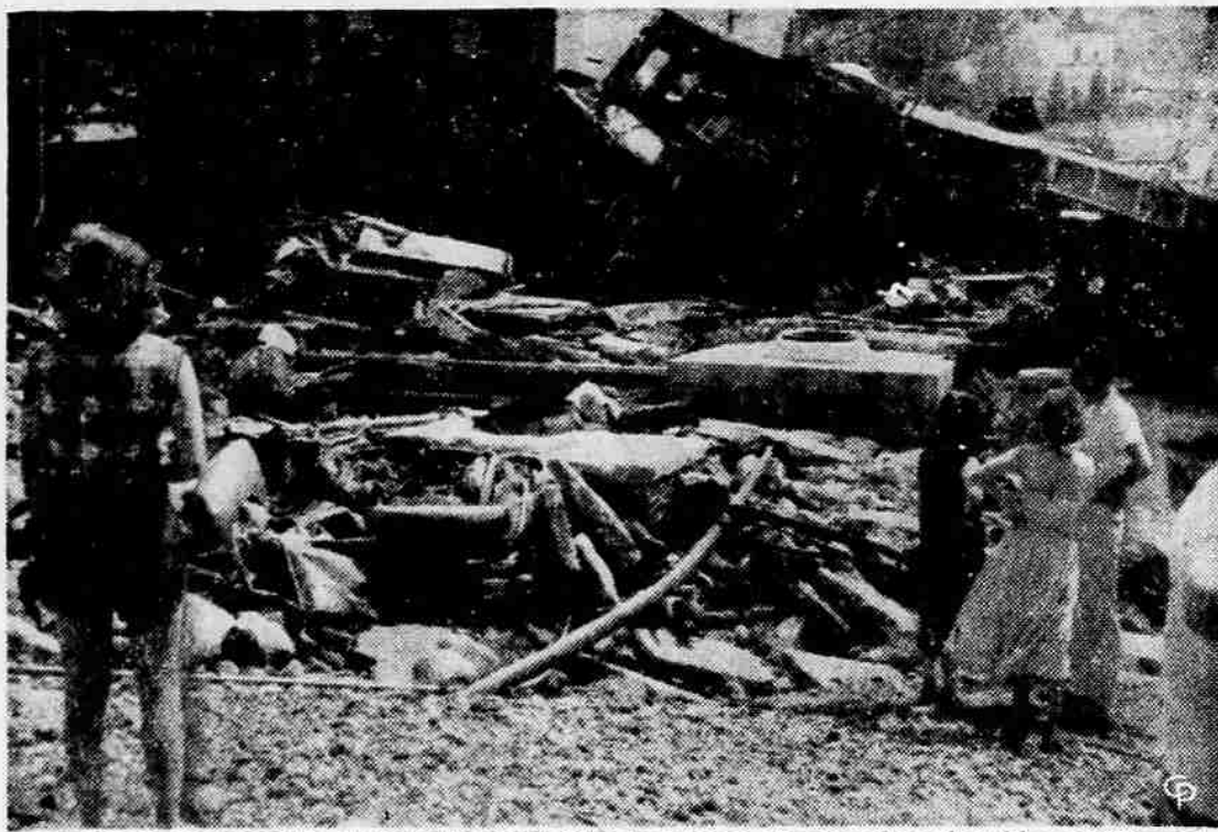
RIPPING THROUGH MAIN STREET like hurricane, flood makes shambles of Winsted, Conn. In foreground left are remains of new sedan. Note two manholes in center, indicating where street level formerly was. In background right is collapsed house. (International)
