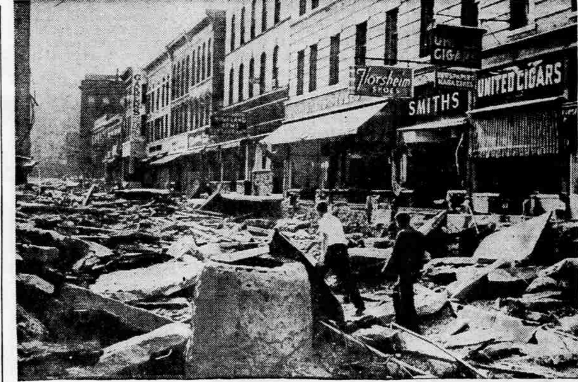
FLOOD AFTERMATH —Main-st, Winsted, Conn., is completely demolished by high flood waters. Two store owners work their way through roadway which was flooded over eight feet leaving only broken water mains and sewer pipes.
