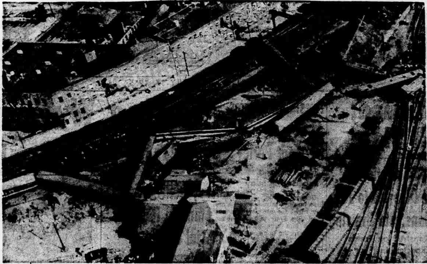
TANGLED 'N TWISTED —At Bridgeport, Conn., a New Haven railroad Washington-to-Boston express train jumped the tracks near the station and went over the banks with the spectacular results shown in above aerial view. One person was killed, 20 injured.
