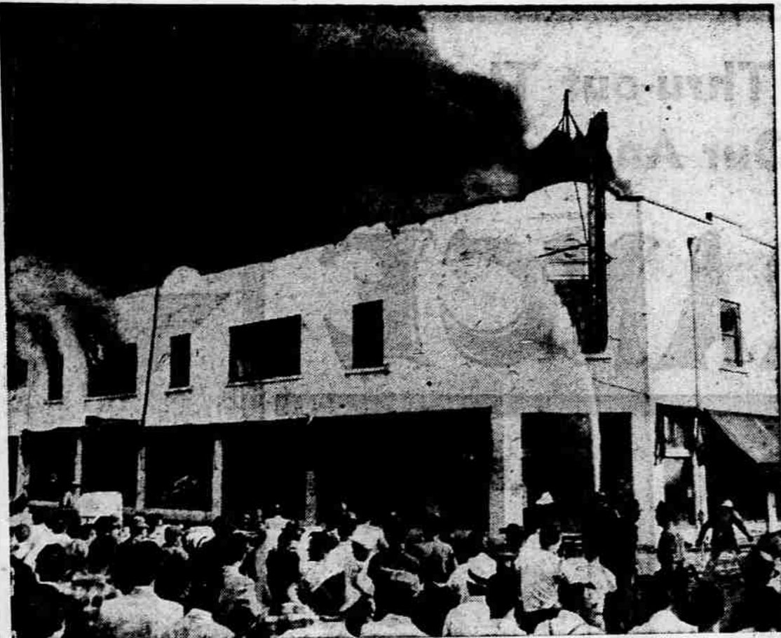
AT HEIGHT OF BLAZE—The fire, which caused damage estimated to be in excess of $100,000 at the Medford Furniture store Friday is shown at its height Friday afternoon. Small at first, it spread rapidly in the upper story, endangering firemen and destroying a considerable amount of equipment. Cause of the blaze has not been determined, but an investigation is continuing.—(Brainerd photo.)
