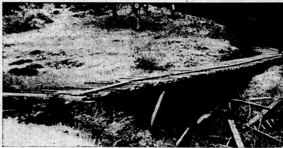
REHABILITATION NEEDED — Another flume carrying water to the valley floor is shown above. It is planned to replace such structures with concrete conduits if next Friday's vote by water-users of the Medford
