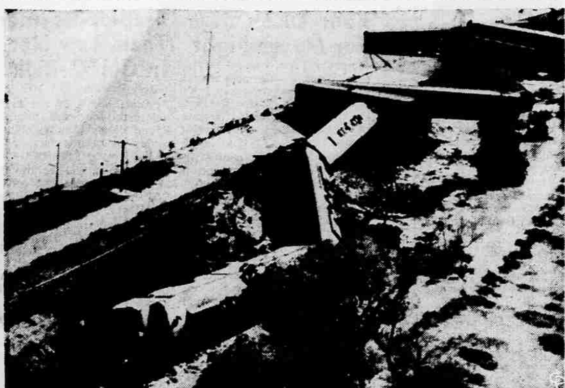
SPRAWLED ALONG right of way, three diesel units, 10 cars are off track near Fort Morgan, Colo., as flash flood undermines rails carrying Union Pacific Streamliner, causing death of train crewman, injuries to 11 passengers. Traffic was tied up many hours. (International)
