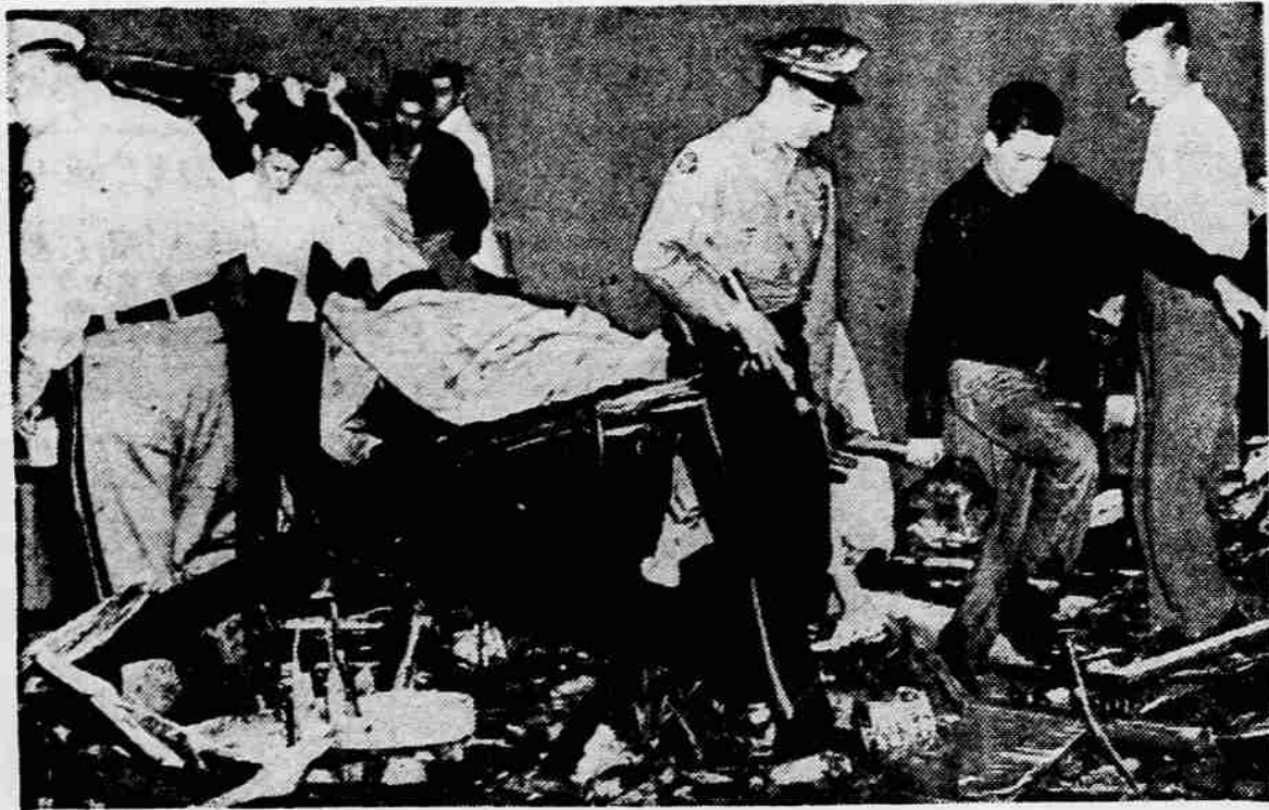
DIGGING VICTIMS OUT —As men in left background hold a wall, rescue workers carry a victim from his tornado wrecked home at Udall, Kas.
