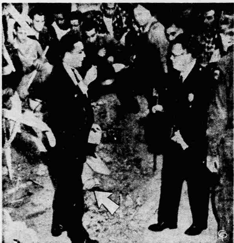
HAND OF VICTIM (arrow), protrudes from wreckage of Coliseum Building, New York, part of which collapsed, as priest and fellow workers pray for him. Joseph Lombardi, 55, was only one of 52 workers periled by crash to lose life. (International)
