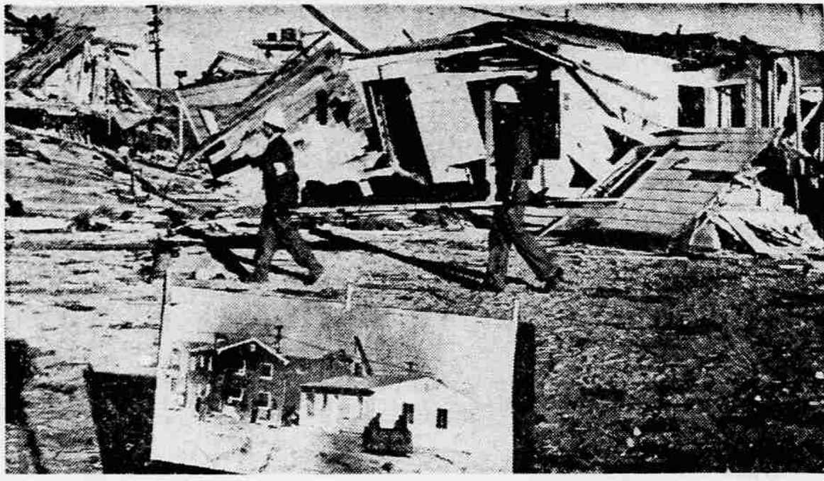
FRONTLINE HOUSES WRECKED BY A-BLAST —Civilian Defense workers remove mannequin "victim" killed by the atomic blast which destroyed his one-story frame house located 4700 feet from explosion in "Survival Town" at the Nevada test site. At top left is seen the Paul Darling two-story brick house which was also destroyed, "killing" the entire Darling family. In foreground is photo showing houses before the blast.
