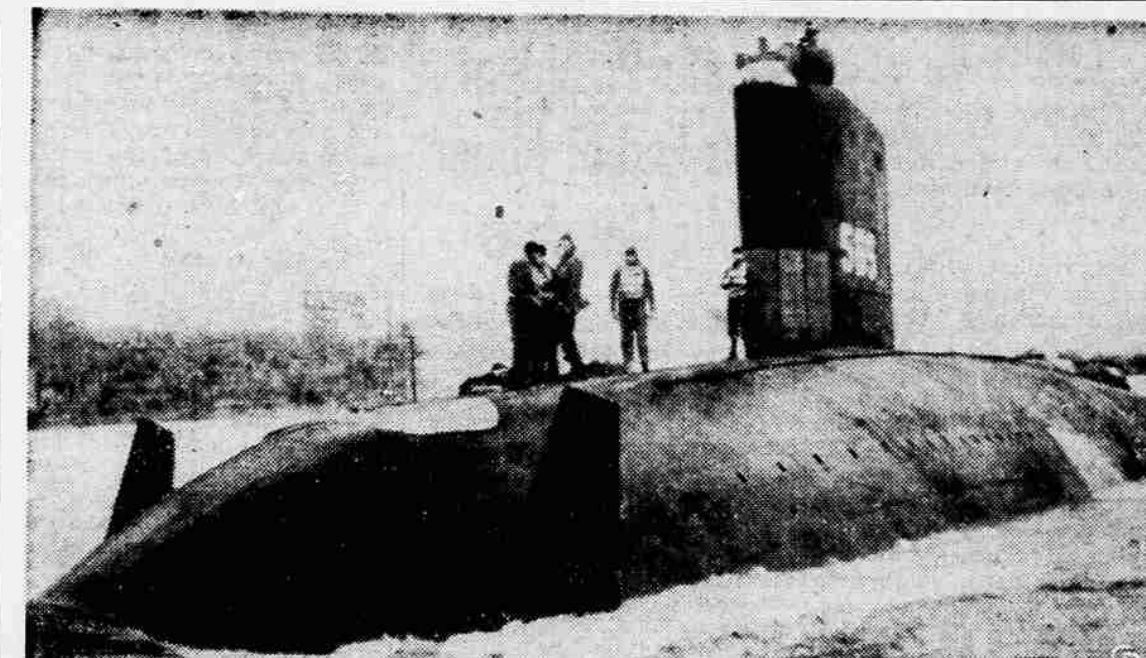
FASTER THAN ATOM-POWERED NAUTILUS under water, this is U. S. Navy's new streamlined submarine Albacore. Its revolutionary design holds superstructure to minimum, eliminating customary flat deck. Experts say atom power would enable Albacore to attain speed of 40-50 knots under water, remain indefinitely at sea. (Collier's Magazine Photo from International)
