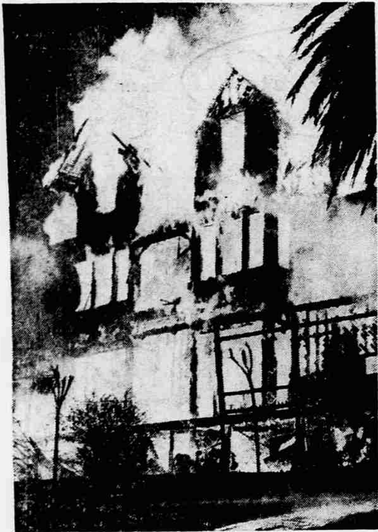
FLAMING FURY —Leaping flames brighten night sky above The Lodge, a three-story rooming house in San Rafael, Calif., which was destroyed in early morning fire, killing at least seven persons. Loss was estimated at $100,000. One tenant is still missing.
