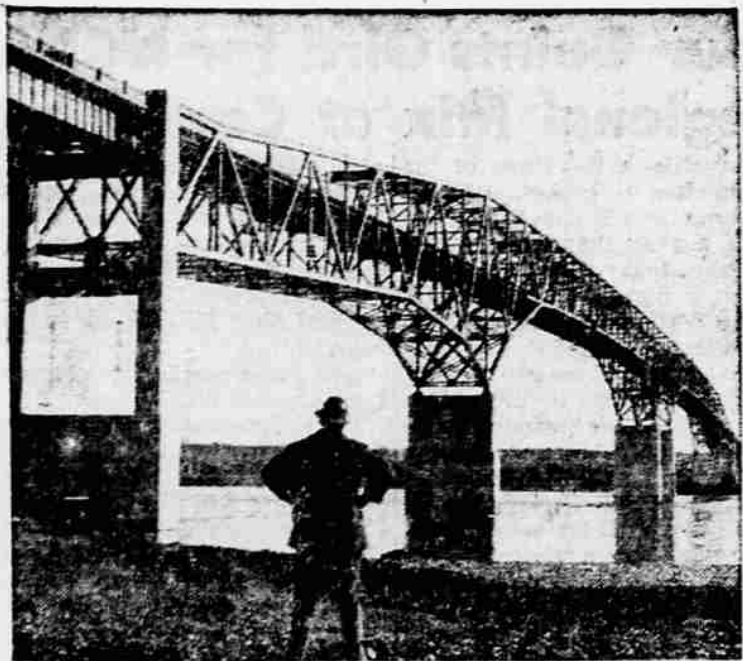
TRAFFIC TIME-SAVER nearing completion in the Northwest is this new span being built by U. S. Steel's American Bridge Division across the Columbia River at Umatilla, Ore., just below McNary Dam. The 3500-ton steel crossing will replace a ferry operated by Umatilla County. It will cut motorists' driving time from Oregon to Spokane and other Washington locations.
