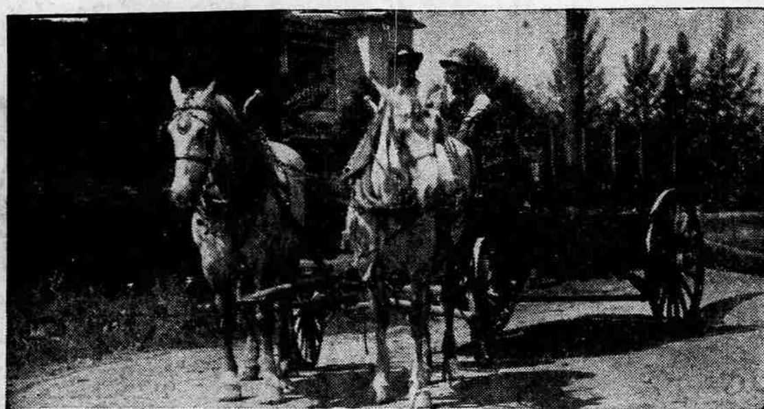
Taken about 1910, this picture shows Grover Medley, now of Joplin, Mo., and Frank Stinson, 311 Vancouver avenue, early-day employees of The California-Oregon Power company. The two men are hauling a power pole with an Eads' transfer team and wagon. Both men are now retired, but Mr. Stinson's son, Lester, is an assistant electrical engineer for the utility. The picture is from the collection of James A. Medley, a brother, 333 West Jackson boulevard.
