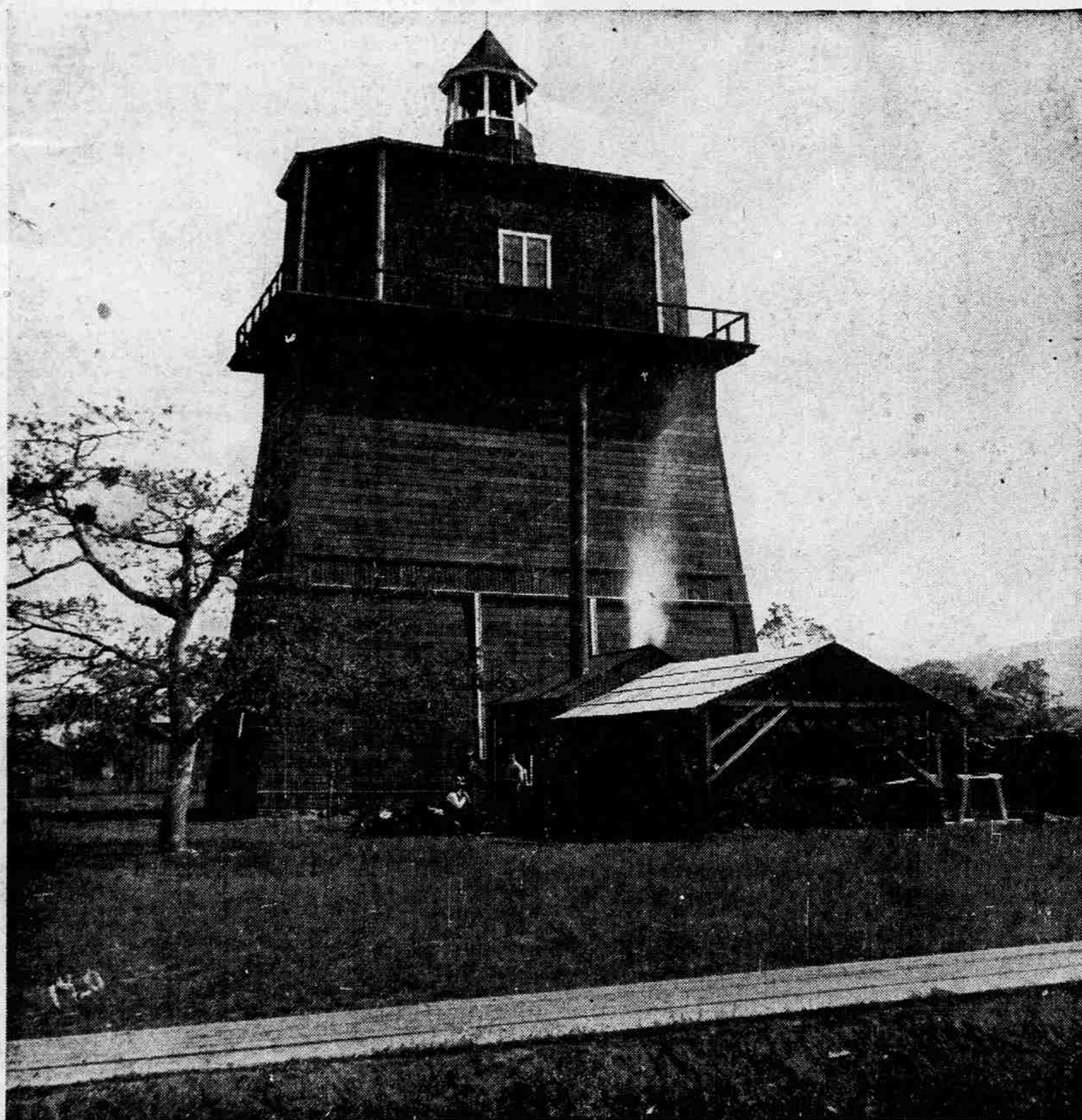
One of the pictures in the collection of Mrs. H. A. Stanley, 35 Crater Lake avenue, is this city water tower which stood where the public library, built in 1911, is now located. According to the "History of Medford" at the library, water was brought in an open ditch from Bear Creek and pumped into two wooden tanks. In 1902 the ditch was abandoned and a pumping plant established on the west bank of Bear creek. Mrs. Stanley's pictures for the most part originally belonged to her uncle, H. G. Nicholson, pioneer Medford merchant. Mrs. Stanley, the former Gladys Curry, is a member of an early-day family and her parents were John W. Curry and Anna Plymale Curry.
