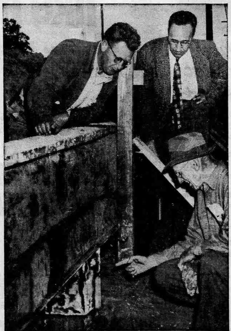
Telephone men use ice to lower cable. To allow for street repairs telephone men had to put this cable deeper in the ground. But they had to lower it very gently so as not to crack its tile conduit, which is costly to replace. After the dirt was dug away, blocks of ice were put under the conduit. As the ice melted, cable and conduit sank slowly into place... undamaged. Ingenuity like this helps us save money, keep your service low in cost. Pacific Telephone works to make your telephone a bigger value every day.
