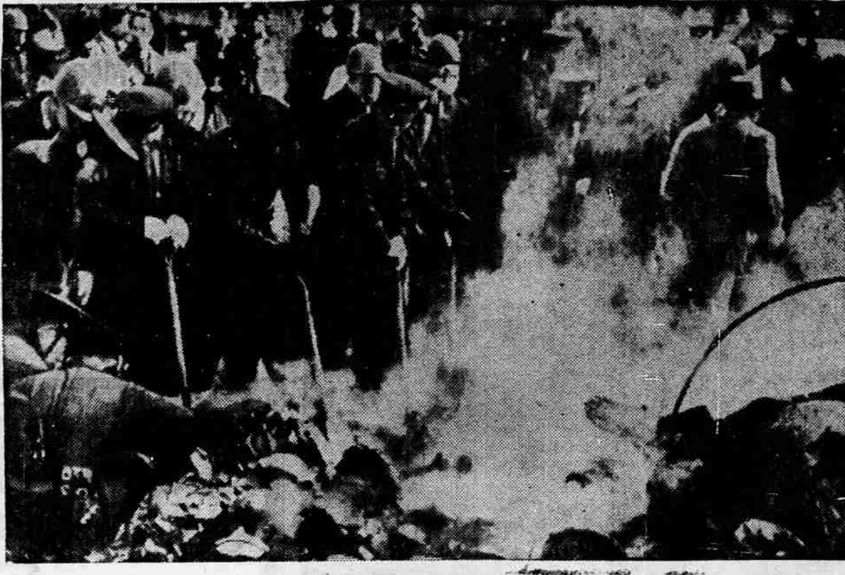
FIRE CLAIMS 99 AGED WOMEN —Police and firemen probe for bodies in the smouldering wreckage of Catholic Mission Home at Yokohama, Japan. Ninety-nine aged women perished when flames swept the condemned structure. Fifty persons, including three nuns, survived the blaze. The two-story wooden building had neither fire escapes or a water supply.
