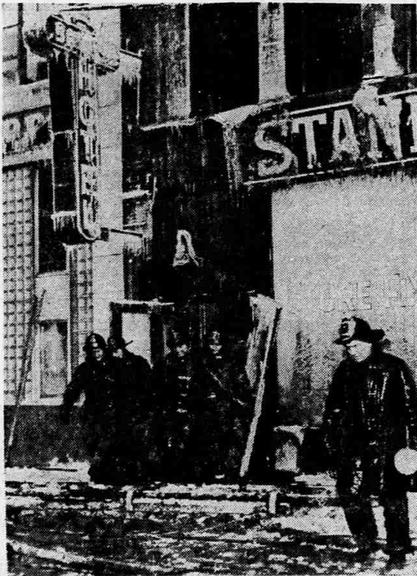
TRAGIC TASK —Ice-coated firemen carry out one of 20 persons killed in an early morning blaze that swept through this five-story hotel on Chicago's skid row. Twelve others were injured in the fire during sub-zero temperatures.
