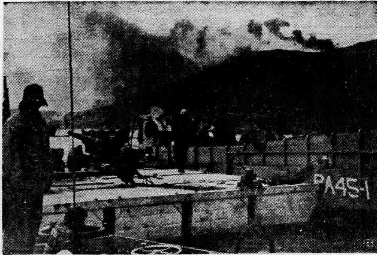
SMOKE RISES FROM INSTALLATIONS on one of Tachen Islands as Nationalist Chinese demolition teams destroy gun emplacements and ammunition supplies before completely evacuating area. U. S. Navy men are watching progress of work to be completed this week-end. (International)
