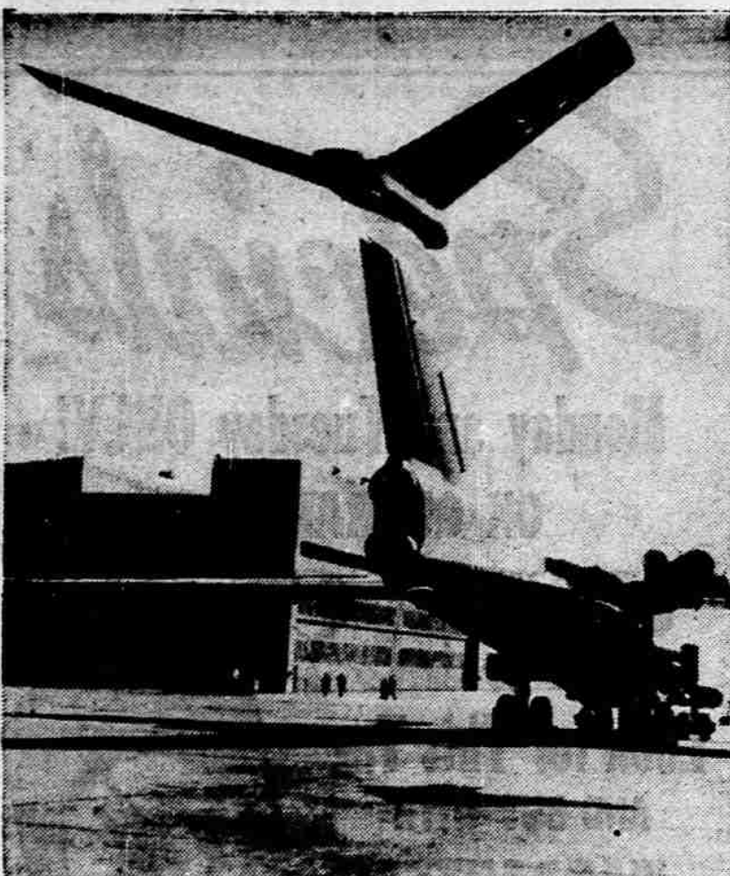
DEADLY PEACOCK —With her sleek tail standing proudly three stories high, the Navy's first multi-jet attack seaplane, the Martin XP6M-1 Seamarbler, rolls out of plant at Baltimore. She is powered by four Allison J-71 turbojet engines and is capable of speeds over 300 m.p.h. The Seamarbler carries a crew of five and will normally cruise at 40,000 feet. The high "T"-shaped tail elevates control surfaces to top of plane's fin to eliminate spray damage.
