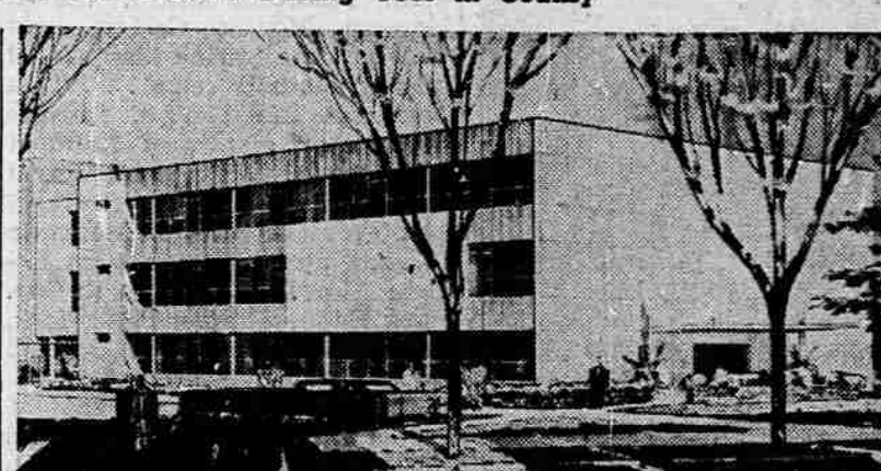
NEW COURTHOUSE ANNEX Construction Started, Progressing
