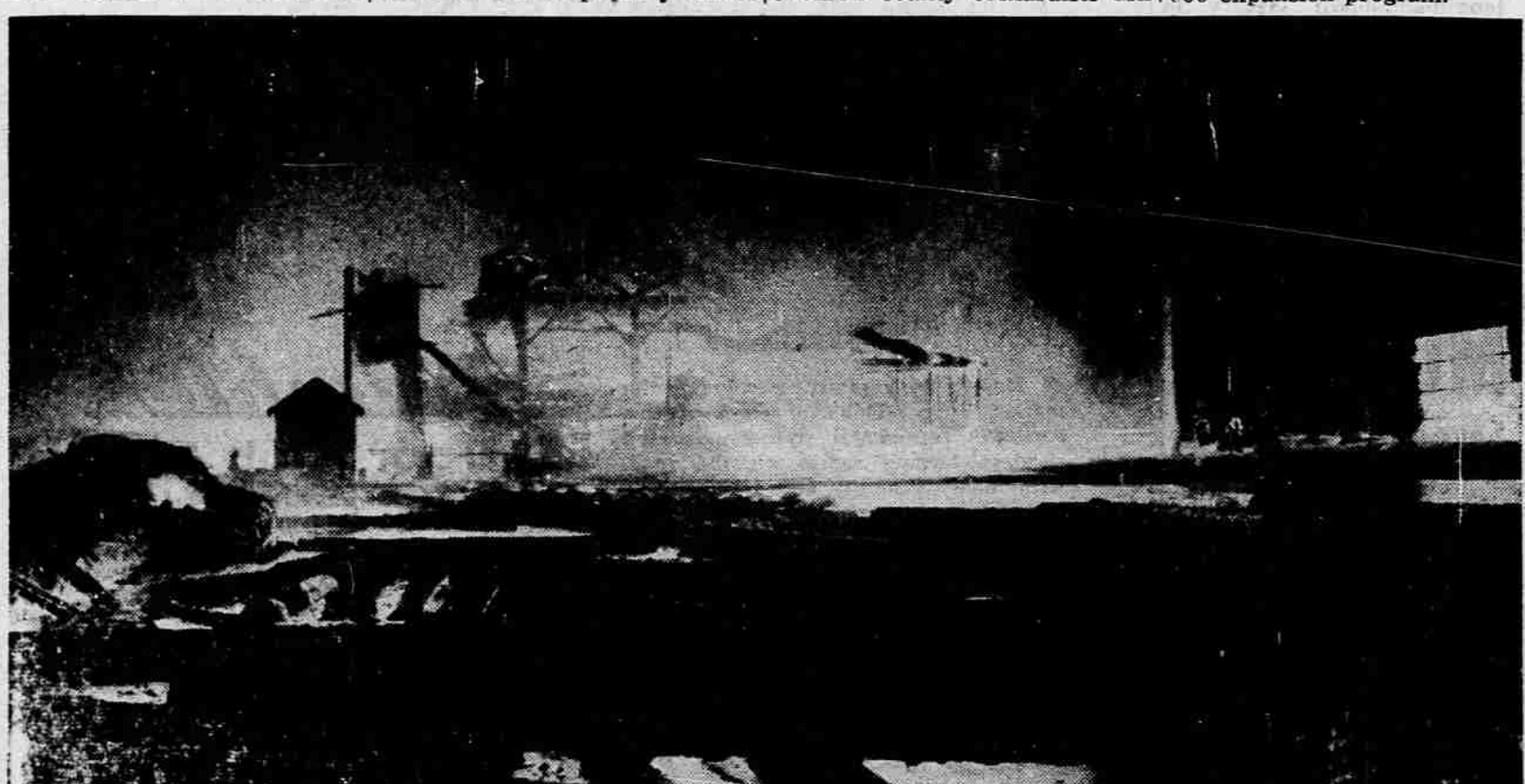
EDMONDS MILL MAKES SPECTACULAR BLAZE SOUTH OF CITY Thousands of Spectators Saw Early-Evening Fire
