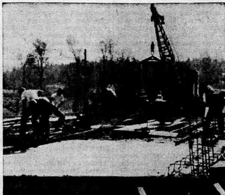
SMOOTHING CONCRETE —Minshall Construction company crewmen are shown above as they smooth cement on the floor of a new bridge spanning Evans creek. The bridge is one of two built at a cost of $23,375.
