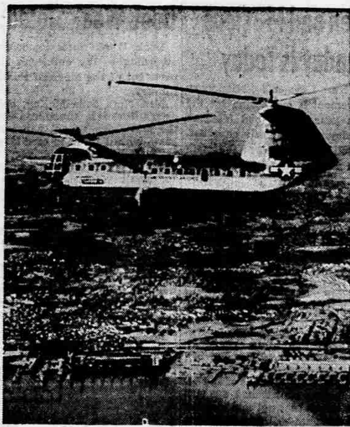
BUILT FOR MORE THAN TWO —The world's largest tandem-rotored helicopter, the Air Force's YH-16 transporter, is shown as it was flown for the first time at altitude. It flew at speeds exceeding 130 m.p.h. and at altitudes of 3000 and 4000 feet over Philadelphia International Airport. The Army will use it for heavy cargo and troop transport.
