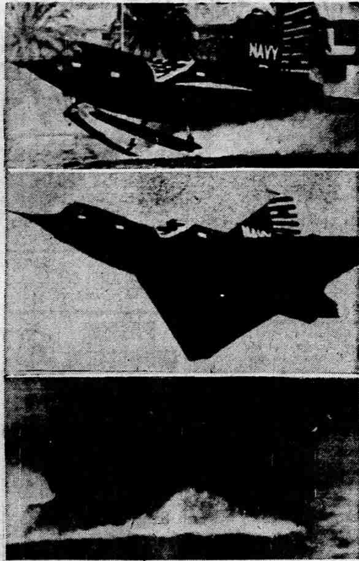
FASTEST JET EXPLODES —Baffled Navy and Convair experts are pressing an investigation to learn why the world's fastest jet seaplane broke up in the air over San Diego, Calif., killing a veteran test pilot, Charles E. Richbourg. In top photo the YF2Y-1 Sea-Dart is shown as it skimmed the water on takeoff. In center it is shown in flight seconds before it exploded. In bottom, wreckage of the Sea-Dart hits the water.
