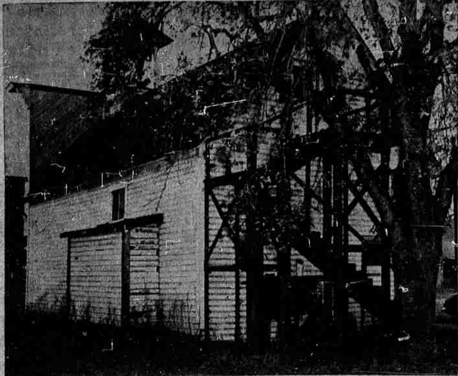
PRESENT FIRE HALL —Pictured is the rear and west side of the Central Point fire hall. The extension on the side was necessary to contain the new fire truck when purchased in 1952. The stairway scaffolding at the rear is considered by Fire Chief Oran Chastain as the
