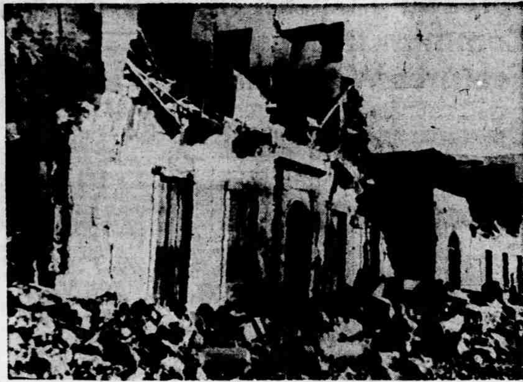
THREE DAYS OF 'QUAKES—Buildings are reduced to rubble and streets strewn with wreckage at Vasshi on the Greece island of Ithaca following three days of earthquakes which ravaged the Ionian Sea islands. Five hundred persons are reported dead.
