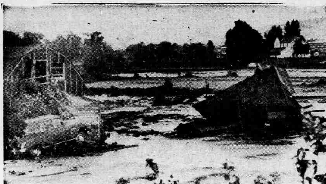
FREAK STORM WREAKS HAVOC —One of two homes swept from their foundations by a flash flood near Yakima, Wash., floats downstream after a freak storm struck the area. A mother and her son are missing in the debris.
