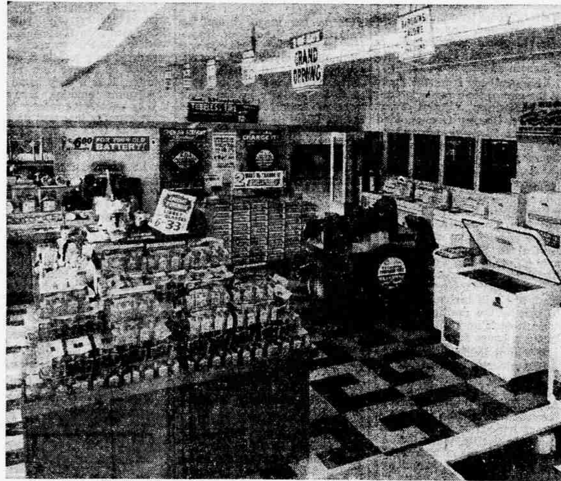
INTERIOR VIEW —Above is an interior view of the Johnston store in Medford, which is observing its first anniversary here this week end. The firm, dealers in B. F. Goodrich products, handles a wide range of automotive and household items.
