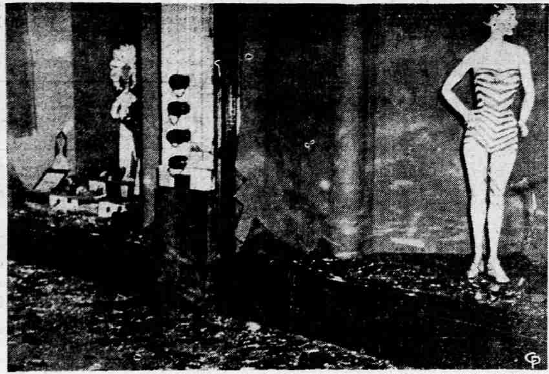
ROCKING SOUTHERN CALIFORNIA, major earthquake causes millions of dollars of damage, much loss of life. Large plate glass windows in Los Angeles' May Company department store are ripped out by temblor which virtually razed town of Tehachapi. (International Soundphoto)
