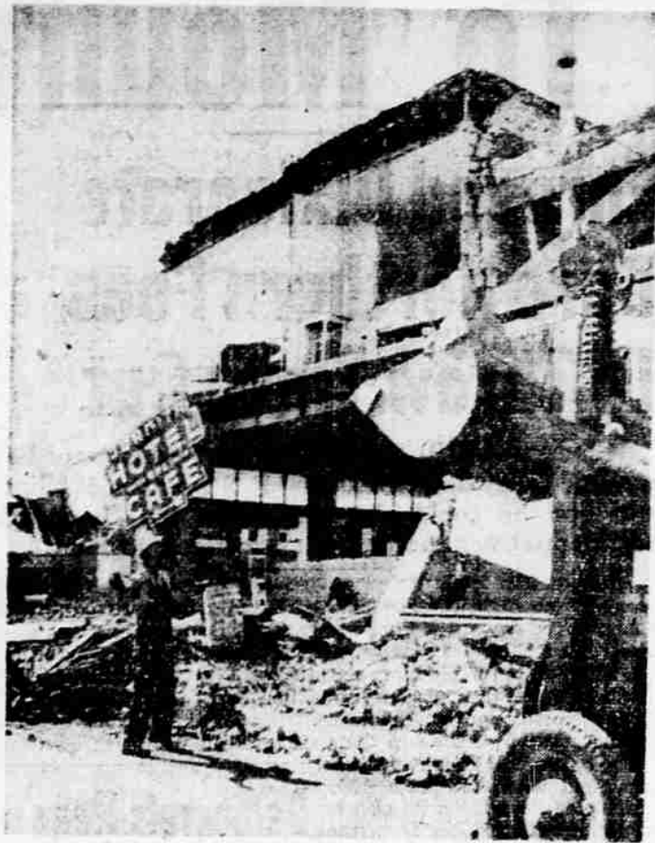
WHERE QUAKE STRUCK —Wreckage of the Juanita Hotel in the tiny Southern California town of Tehachapi, where at least 11 persons died in a severe earthquake that was felt over nearly 600 miles of California. It was one of the severest in state's history.
