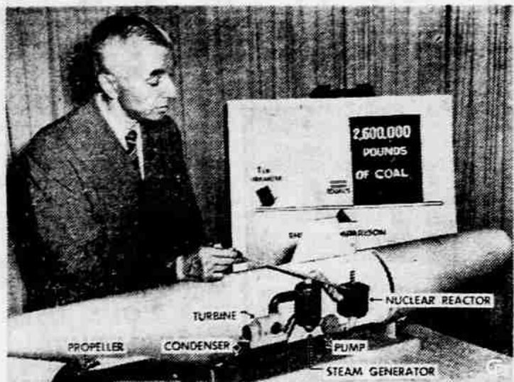
USING MODEL of atomic submarine, Capt. Hyman G. Rickover, Navy's nuclear power expert, explains how it operates. Heat is created in nuclear reactor by fission of uranium. This heat is transferred to steam generator which drives turbine from which power is transmitted to propellers. Craft has enormous range (International)
