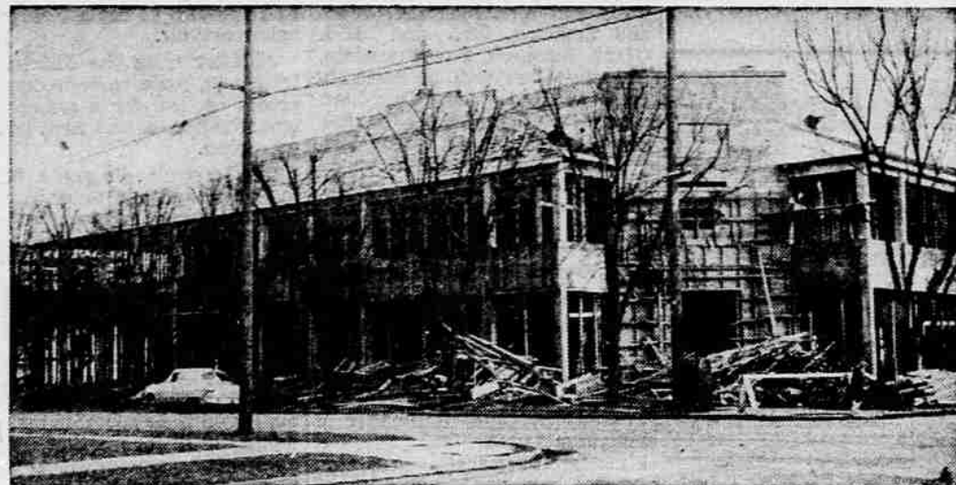
OLD BUILDING TO DISAPPEAR —The picture above, taken during the construction of the new St. Mary's school building, also shows the old building looming above and behind the new. The old structure will soon be demolished, after serving the academy and the school since 1908. The modern new school building was constructed in an L-shape around the old building.
