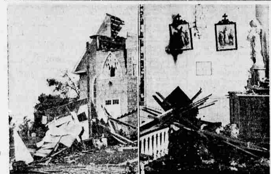
BUFFETED BY NATURE —St. Jeanne's Catholic Church at Corcoran, Minn., fell victim to heavy winds during a two-day storm. The roof and steeple (left) were ripped off. Inside the church was covered with debris, but left a Madonna and Child statue untouched. The storms caused heavy damage throughout the state.
