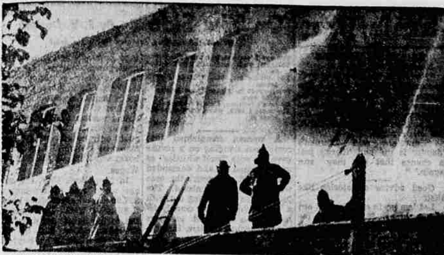
WITHOUT WARNING —Firemen atop adjacent building pour water on the blazing Terre Fiber Box factory in Chicago just moments before this brick wall collapsed on them. At least 12 firemen were injured. The victims were treated for injuries which included broken legs and arms and skull injuries. Fire damage was estimated at $200,000.
