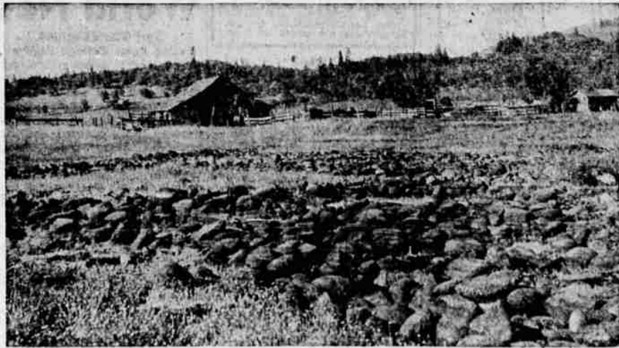
BEFORE AND AFTER IN PROGRAM —Shown above is an illustrative example of the practice of preparing land for irrigation. Pictured (left) is a portion of a 50-acre tract which, according to estimates by the Jackson county extension service, was only supporting five or six head of cattle for a period of two months. After the project was okayed for federal assistance, which was limited to 50 per cent of the cost or $15 an acre, under the Agricultural
