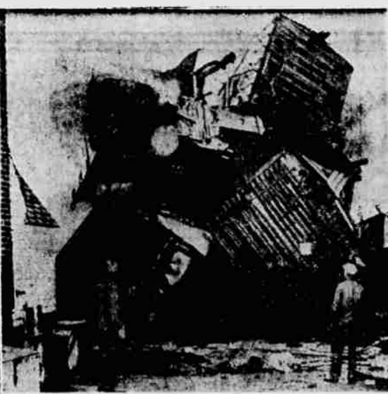
LIKE CORDWOOD —These freight cars, piled one on top of the other, are part of 30 cars of a 60-car Monon freight train that were derailed at Lowell, Ind. Alcohol in six cars burst into flame and threatened the entire business section before being brought under control. No one was injured in the accident.
