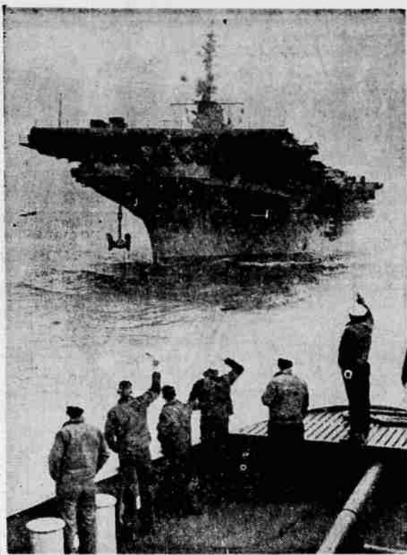
COLLISION SCARS REMOVED —Crewmen of the tub Penobscot (foreground) wave as the aircraft carrier Wasp, fitted with new 90-ton section of bow from her sister carrier Hornet, heads for Gravesend Bay after leaving drydock at Bayonne, N. J. Ten days of round-the-clock repairs removed scars of ship's collision with the destroyer Hobson.
