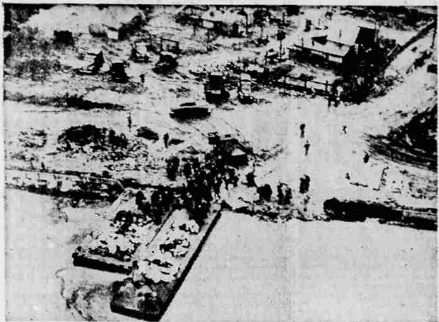
RIVER POUNDS OMAHA DIKES—Army barges bring in sandbags to bolster the levee protecting Omaha, Neb., from the flooding Missouri River. Levee workers saw what white men never had seen before—the Missouri surging past at 30.22 feet. Rain turned the area into a sea of mud.
