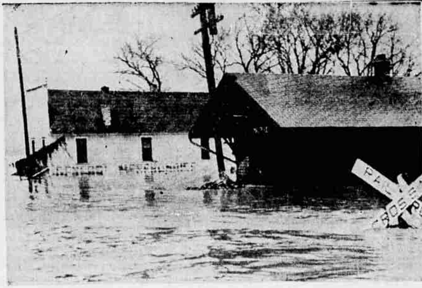
THERE'LL BE NO TRAINS TODAY—Railroad station at McPaul, Ia., was inundated when the Missouri River ripped a 150-foot channel through the nearby Plum Creek levee.
