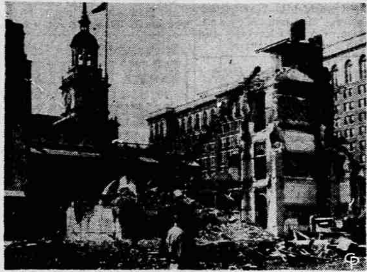
DEMOLITION OF OLD BANK BUILDING is nearly complete, providing better setting for Philadelphia's Independence Hall, most famous American shrine. Historic structure has been partially obscured during years by financial institution. (International)
