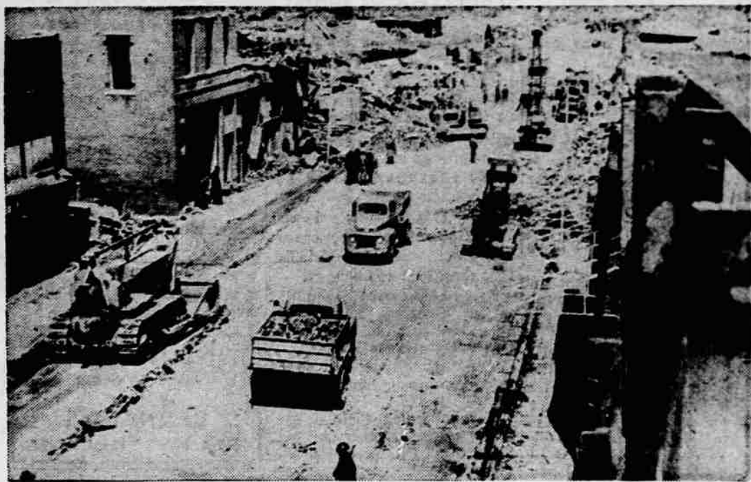
TORNADO-SHATTERED —Heavy equipment rumbles through the streets of Judsonia, Ark., as the community begins the grim task of rebuilding after the greatest barrage of tornadoes in 20 years swept the mid-South. Arkansas, hardest hit by the killer twisters, counted 149 of 250 dead and 711 of 1107 injured.
