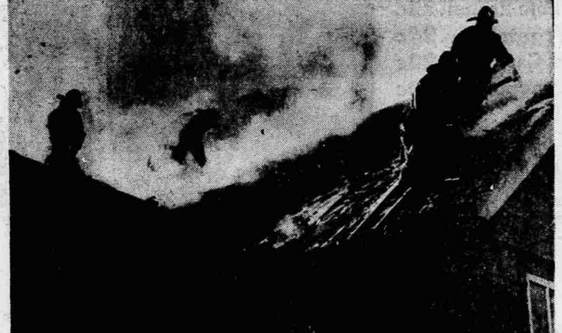
EARNING THEIR NICKNAME—These smoke-eaters are really earning their famous nickname as they crawl on the roof of a two-story Minneapolis house in an effort to put out fire which left 17 persons homeless. All the occupants escaped without injury.
